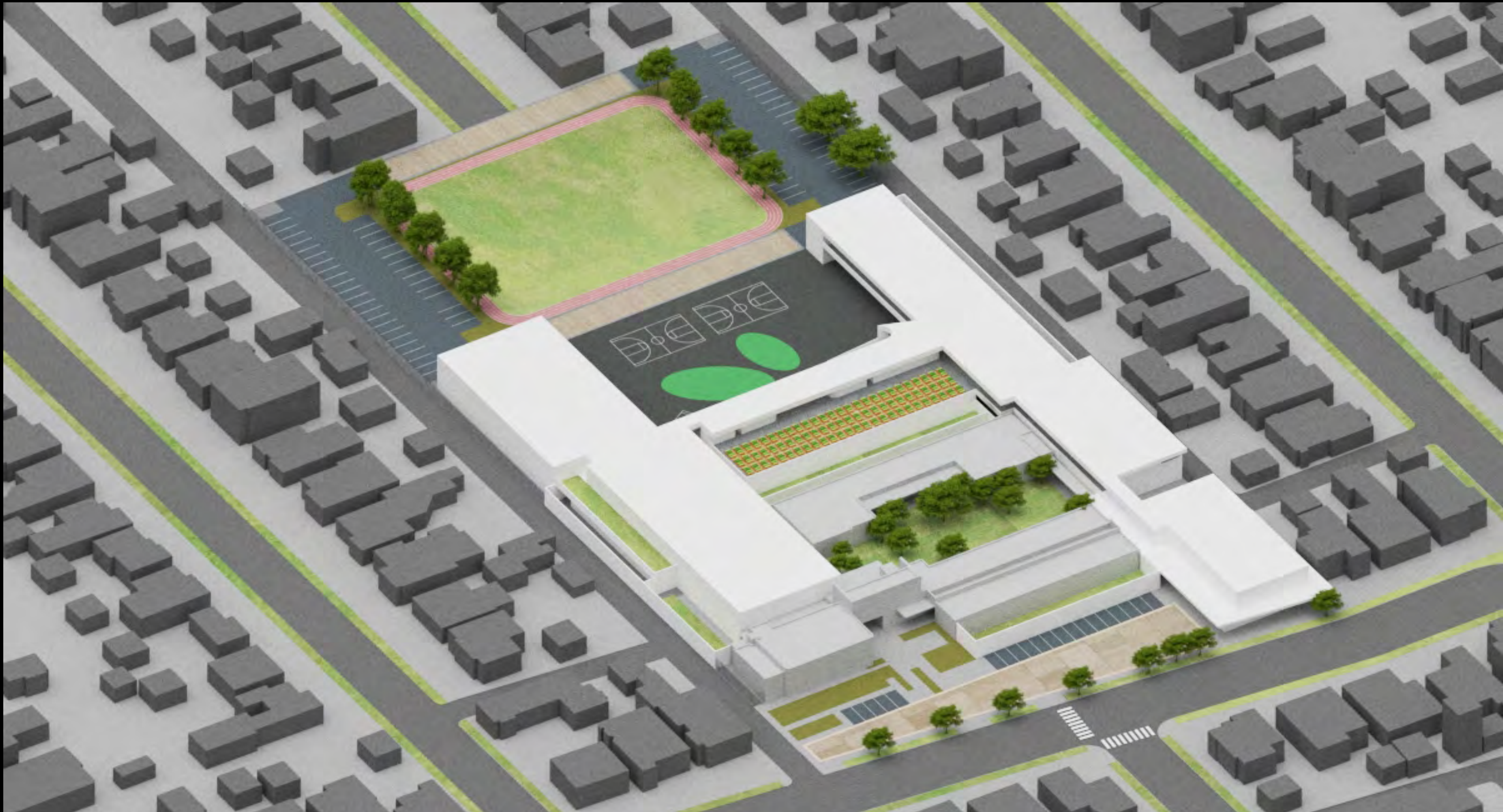
CAMPUS AT COMPLETION
