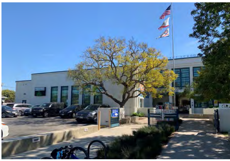
FRONT OF SCHOOL AND AUDITORIUM
